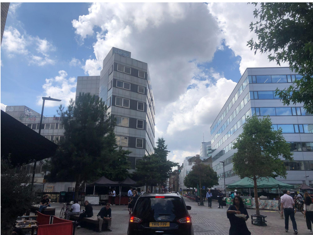
View west over Leonard Circus, of Development House (left) and Telephone House
