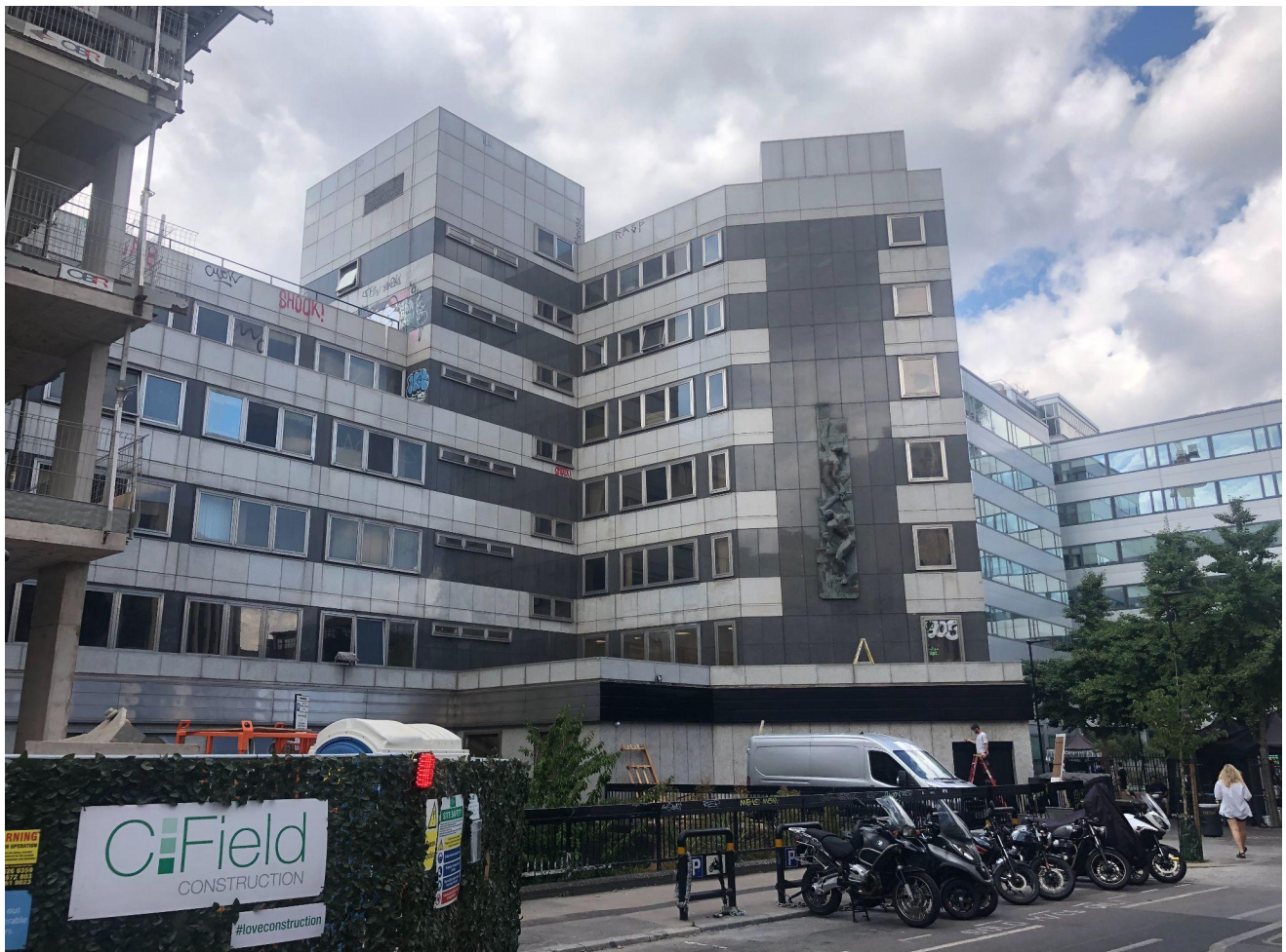
Development House from Paul Street:
